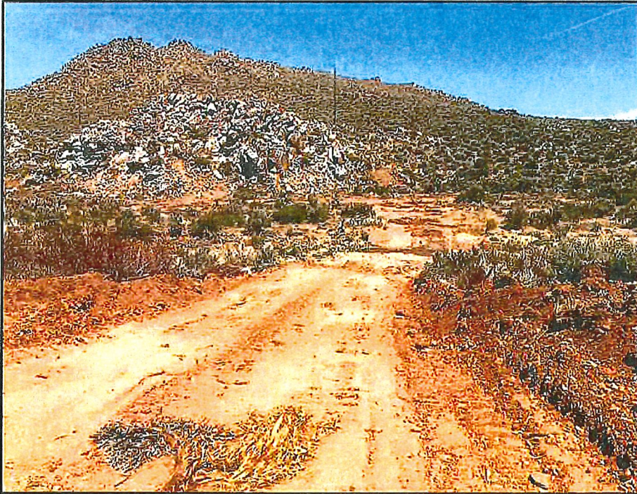
Portion of new access that was "graded" to get across a steep slope on west side of drainageway.
